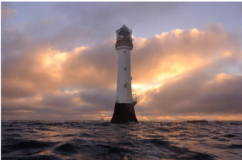
Bell Rock Lighthouse, Skotland
